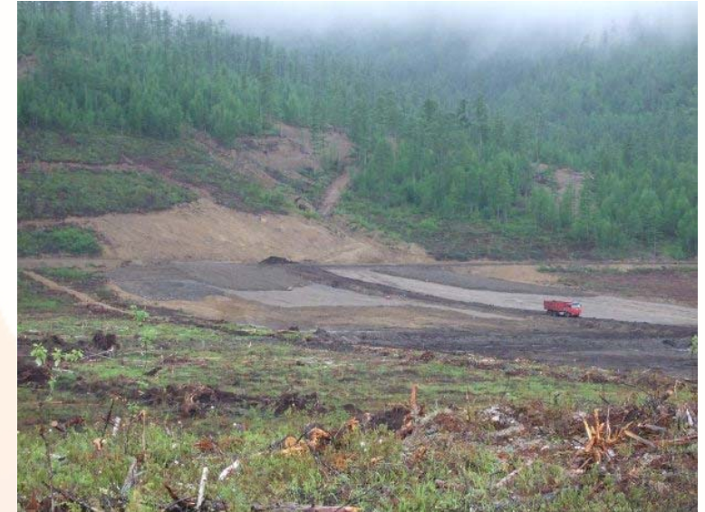
Tailings dam construction
