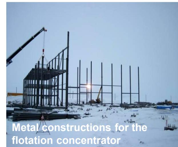
**Metal constructions for the flotation concentrator**
