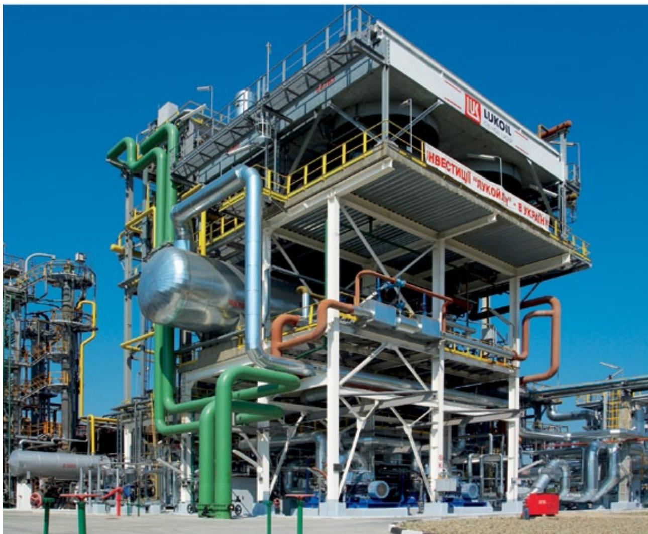
technology. Annual capacity of the new unit will be 182,000 tonnes of gaseous chlorine and 200,000 tonnes of caustic soda. The new capacities will enable Karpatneftekhim to produce caustic soda, which meets international quality standards, and to fully provide the plant's own chlorine needs. Commissioning of the unit is scheduled for the end of 2009.
