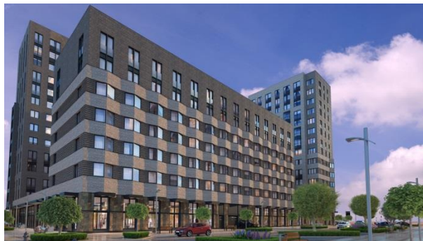
ZILART Land plot – 65 ha Total NSA – 979 th m 2 Start of pre-sales – Sep 2015 Completion – 2025
