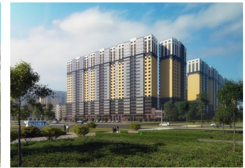
CIVILIZATION Land plot – 60 ha Total NSA – 824 th m 2 Start of pre-sales – March 2016 Completion – 2026
