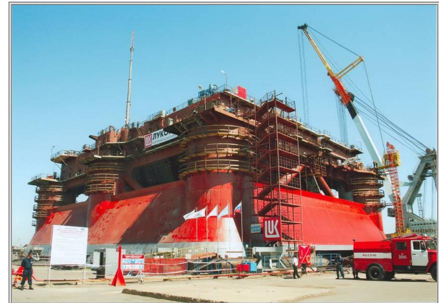
Construction of an offshore platform to develop Yu. Korchagin field.
