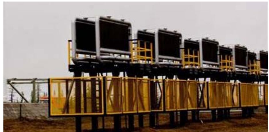
Thermal stabilization of soil
