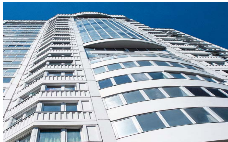
Malomoskovskaya street, Moscow (completed)
