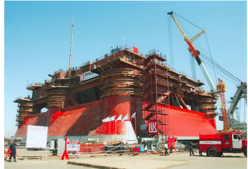
Start of construction of an offshore platform for Yu. Korchagin field.
