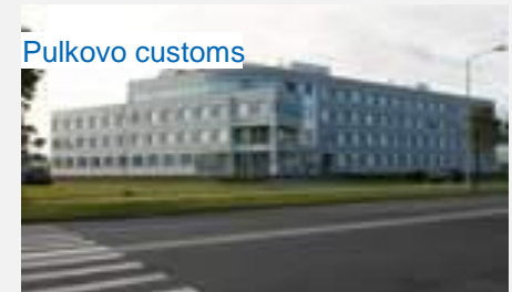
Full construction cycle
